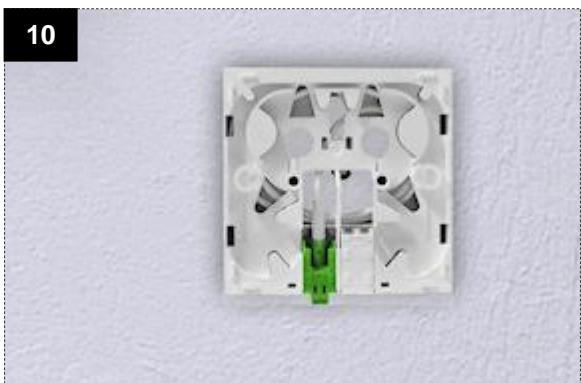
Turn the socket back over and attach it to the metal frame. Be careful to not pinch down the cable.
