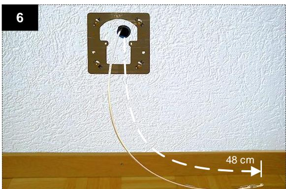
Attach the mounting plate to the wall with four screws.
