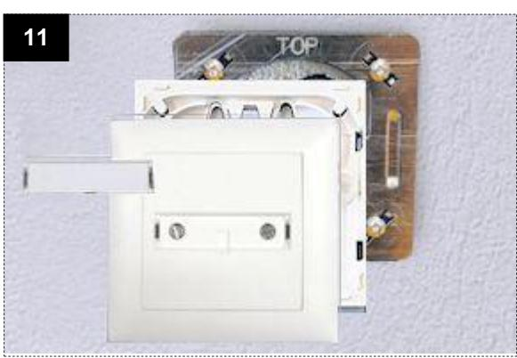
Screw the frame and the cover plate down to the mounting plate.
